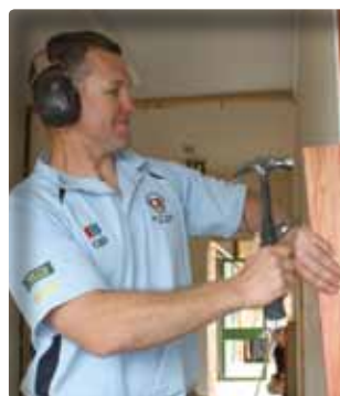
Mark Todd of Absolute Build fits a stud before lining the library walls.
